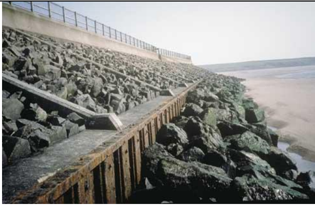
Figure 1c: Groynes to protect the beach (Source: EUCC - The Coastal Union. Copyright EUCC-Deutschland) Source: OSPAR Commission, 2009
