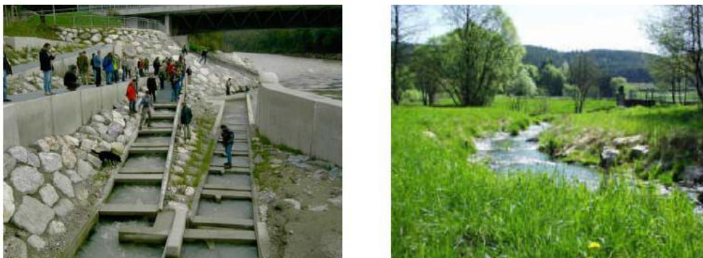
Figure 3: Two types of functioning fish passes – the more natural- like bypass channel is more costly in this case but provides useful additional spawning ground.
