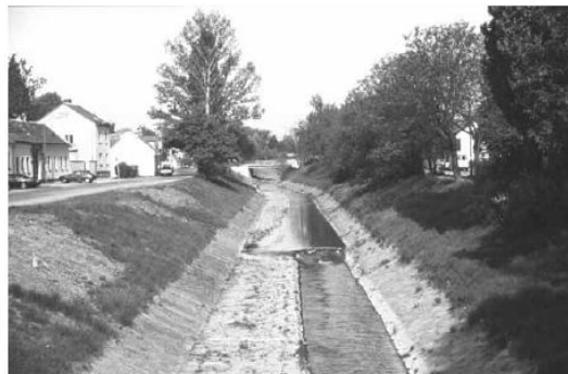
Figure 2. After the flood in 1954 the Liesing was pressed into a u-shaped concrete bed.
